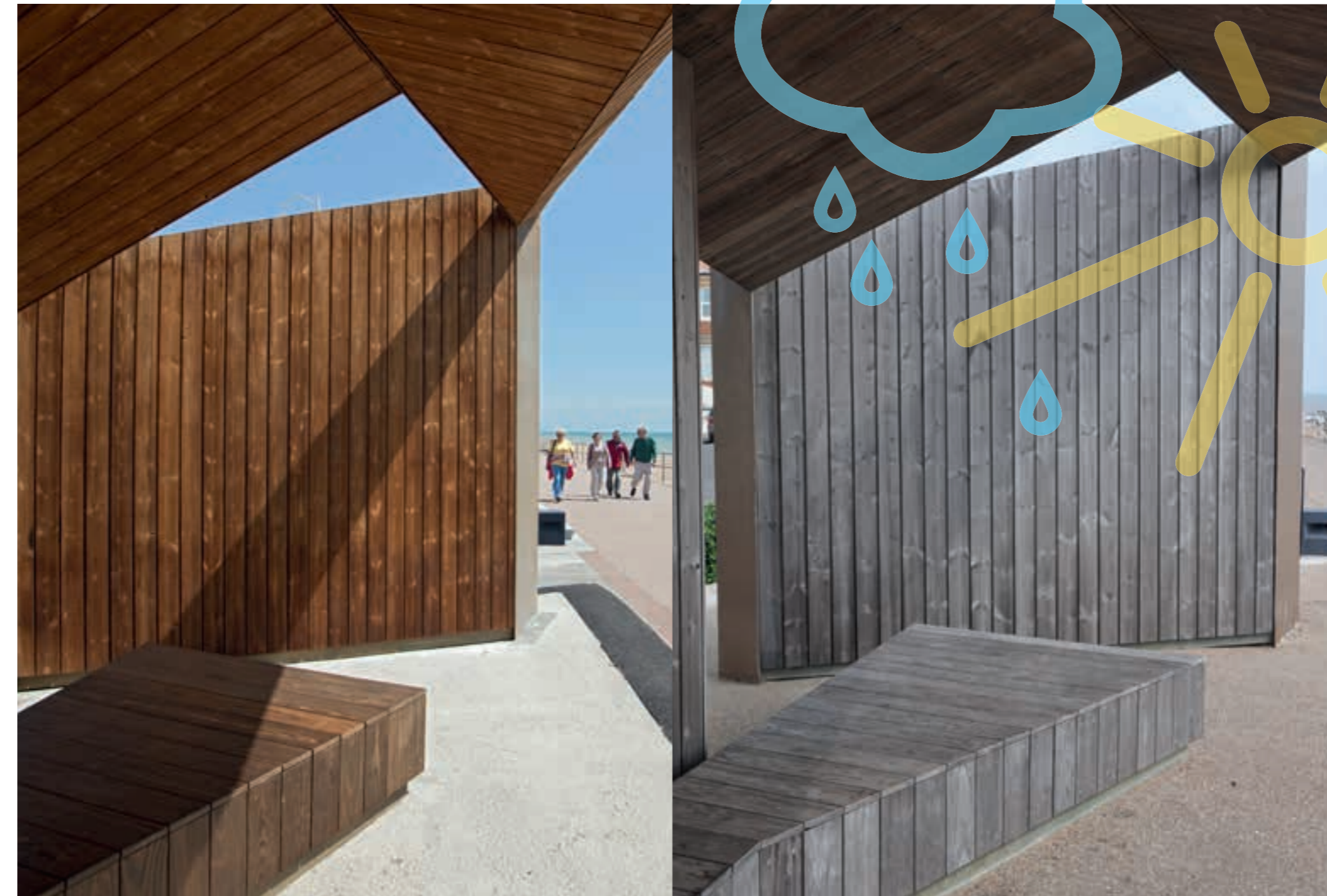
The Beach Pavilion Bexhill-on-Sea in Sussex / UK. The pictures show how the elements have given the wood a beautiful patina. Below left: NEW WOOD. Right: WEATHERED.
